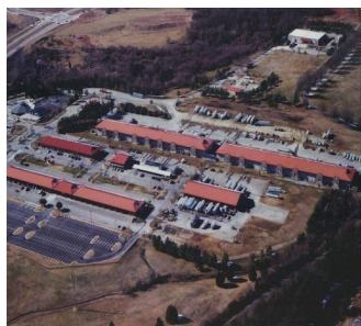
This existing Raleigh State Farmers Market will be redesigned under a master plan. Courtesy of North Carolina Department of Agriculture
