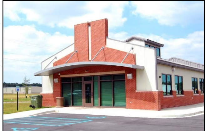
New Administration building
